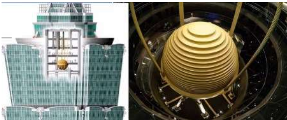
Tuned mass damper of Taipei structure
