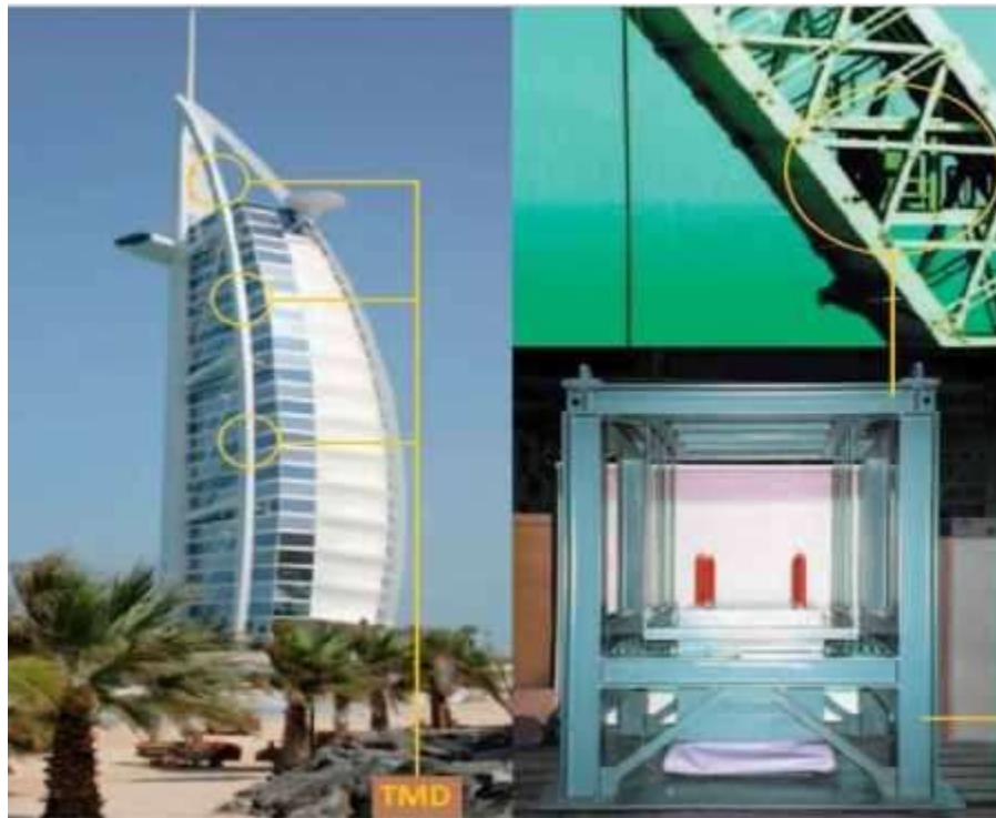
Tuned mass damper of Burj Al Arab
