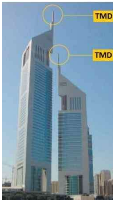
Tuned mass damper of Emirate tower
